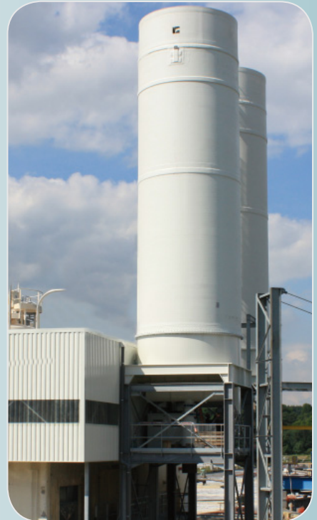
○ Twin silos, 2 x 240 m 3 with building extension (ADISSEO).
