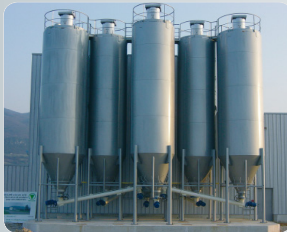
6 Silos Ø 2500 mm capacity 50 m 3 (CAMPENON)
