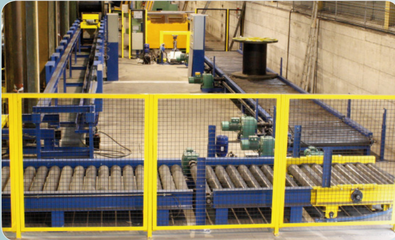
Steel wire coil circuit (ACOR)
